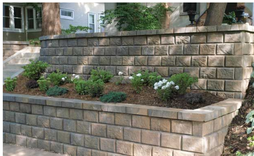
Retaining Walls: Allan Block Fieldstone Sierra Series Color: Rustic Creek or sim.
