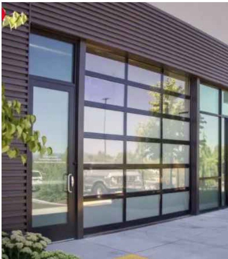
5 ALUMINUM AND GLASS ROLL-UP DOOR CLEAR GLASS SET IN BRONZE FRAMES TO MATCH #3 ALUMINUM CLADDING
