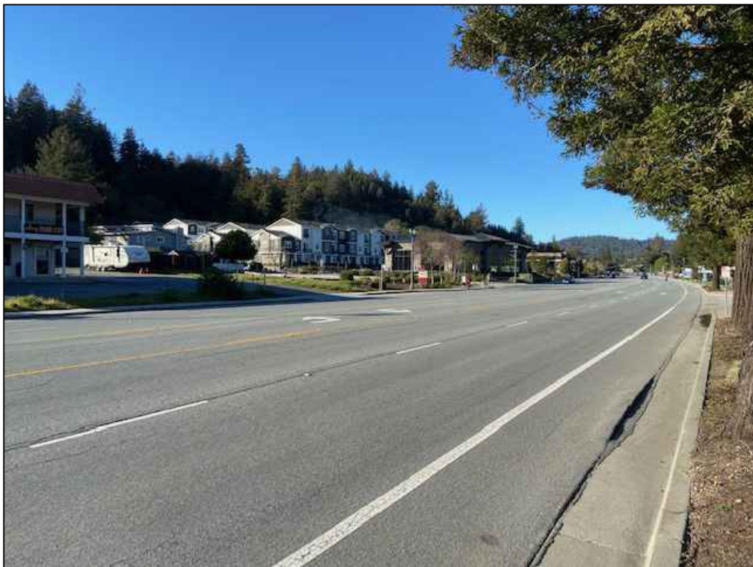
D VIEW LOOKING NORTH ALONG SCOTTS VALLEY BOULEVARD
