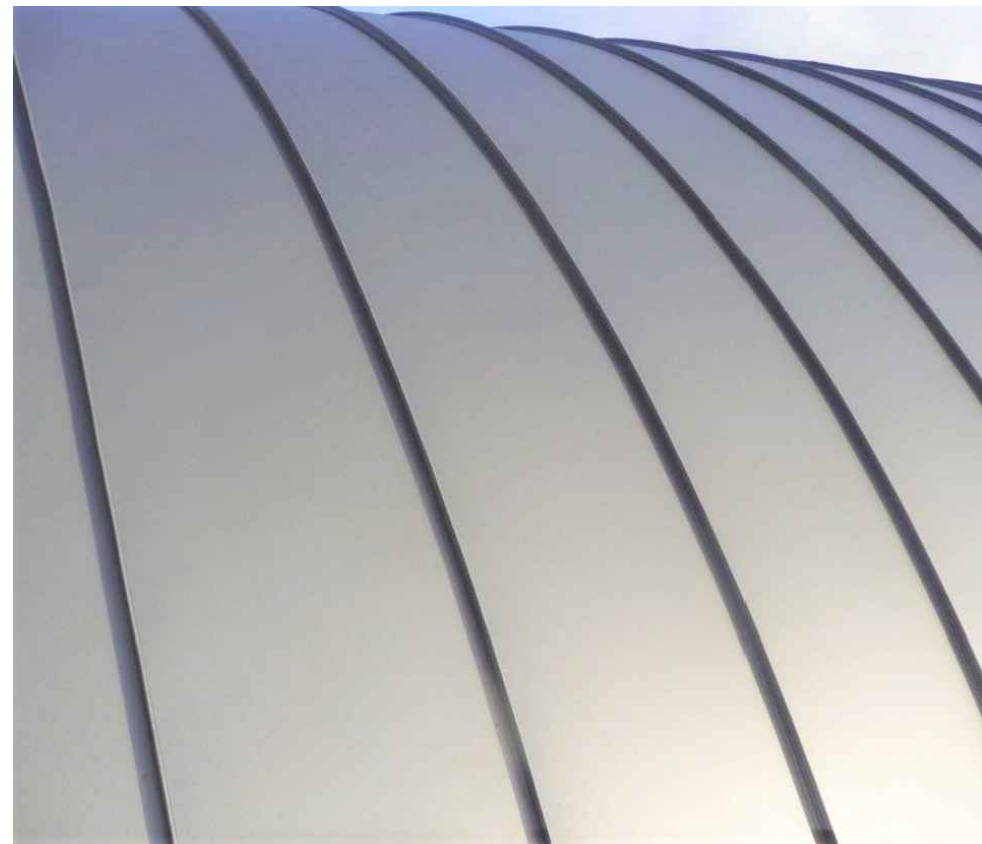
8 ALUMINUM RIBBED ROOFING (NATURAL ALUMINUM COLOR)
