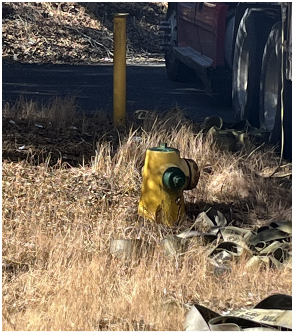
5 EXISTING FIRE HYDRANT LOCATION: SOUTHEAST CORNER OF SITE
