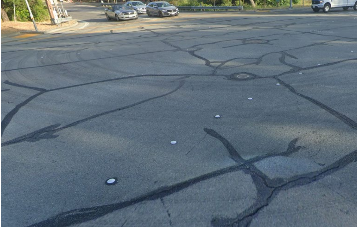
Pavement cracks along Scotts Valley Dr
