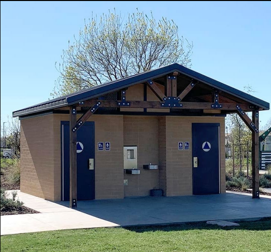
Pre-fabricated concrete restroom building
