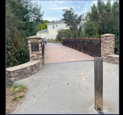
Existing bridge stonework and weathered steel members, inspire material and finishes
