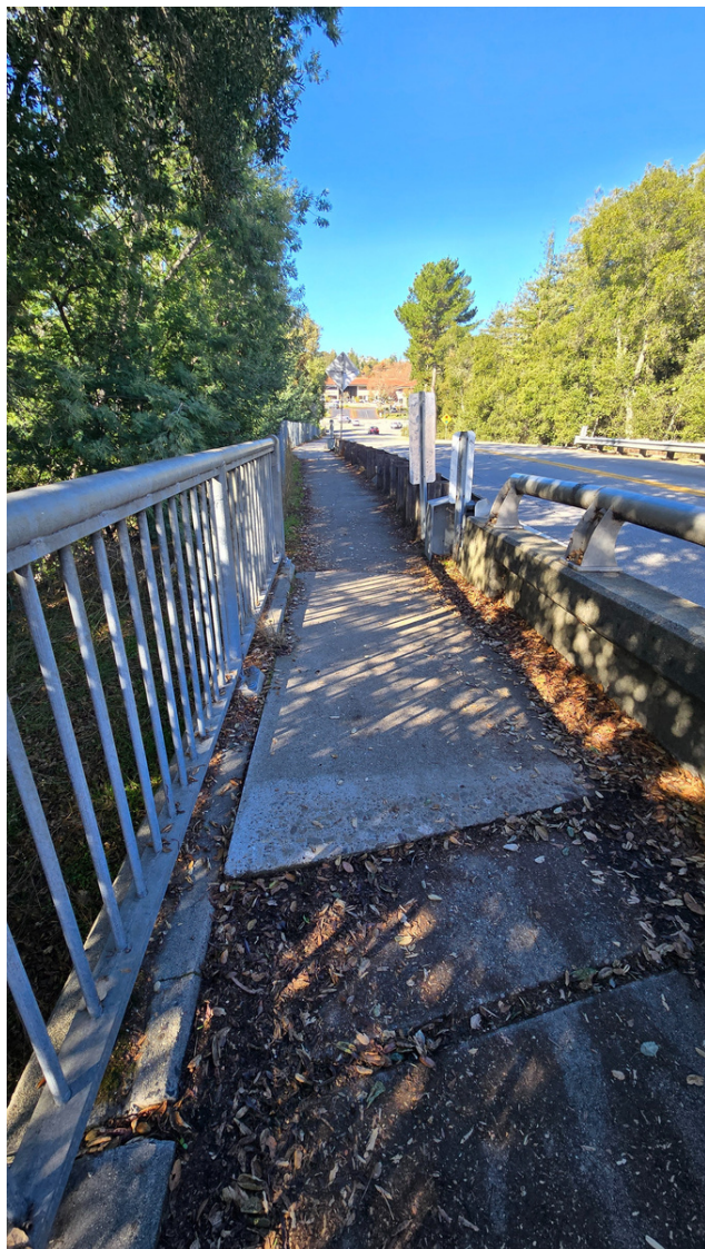
Exhibit E: Granite Creek Overcrossing Guardrail and Pedestrian Walkway Towards Santa's Village Road
