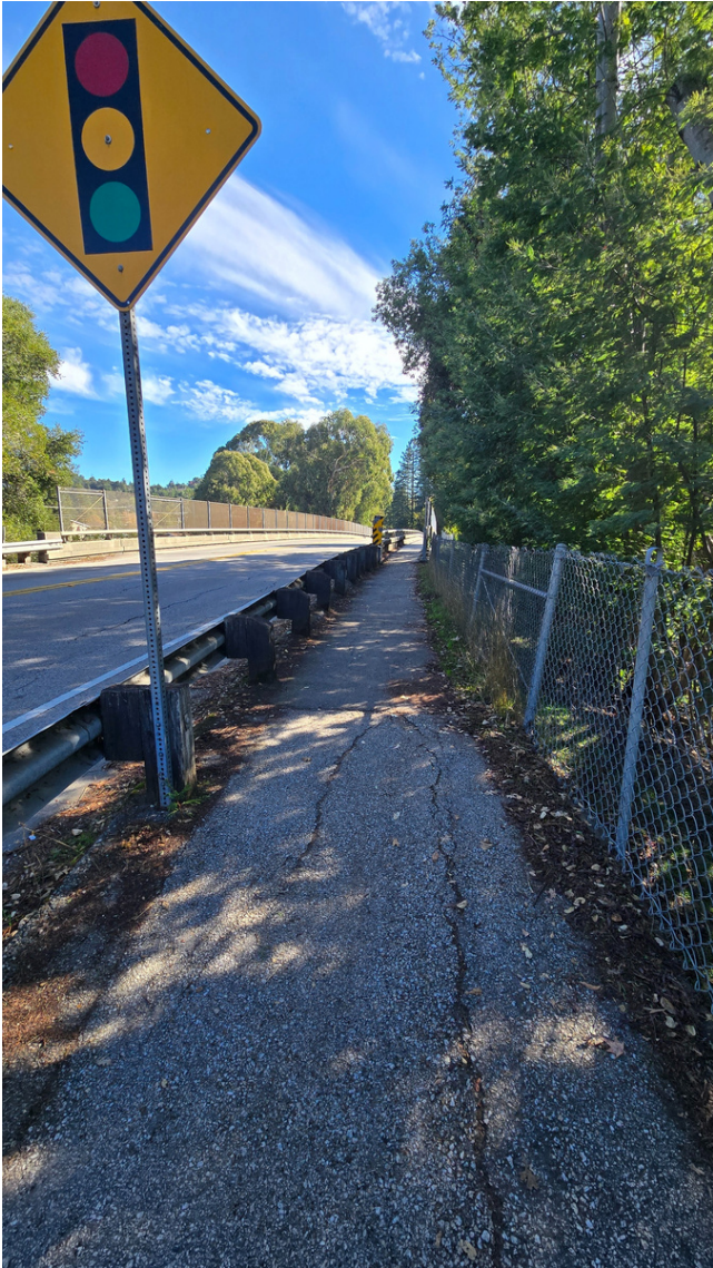
Exhibit C: Granite Creek Overcrossing Guardrail
