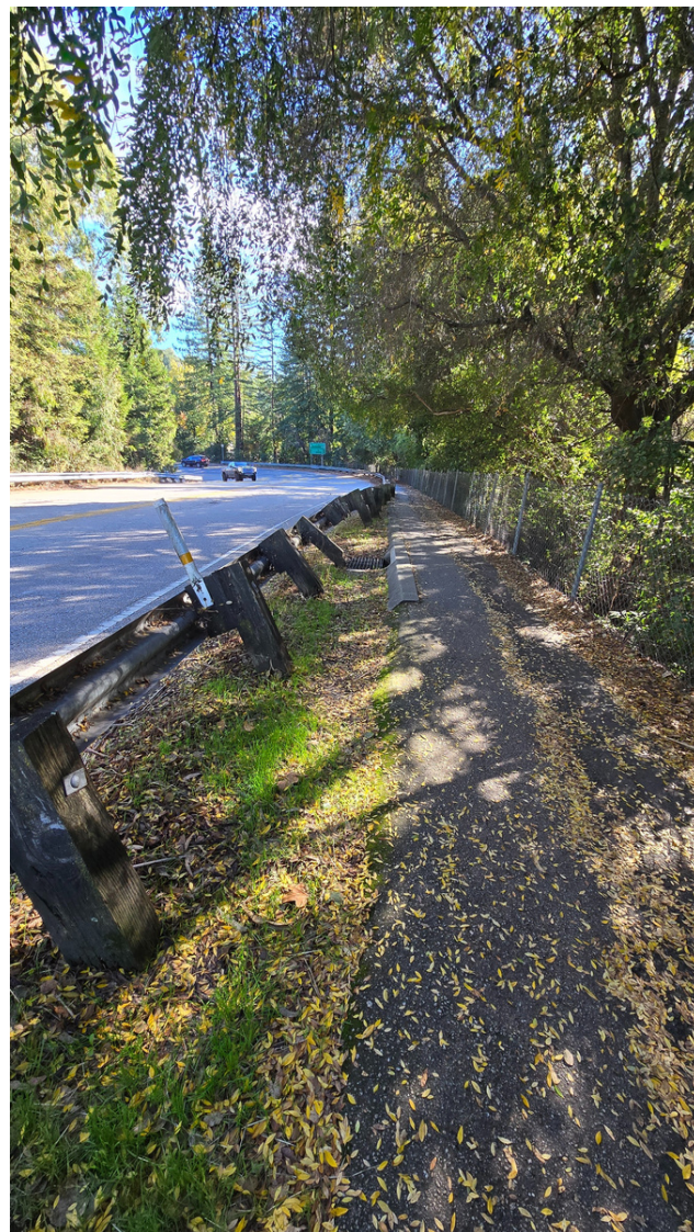
Exhibit F: Granite Creek Overcrossing Guardrail and Pedestrian Walkway Towards Santa's Village Road
