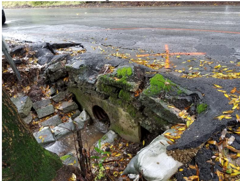
Drainage Failure 1/17
