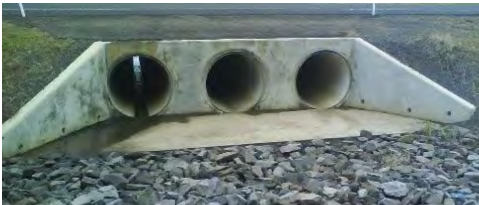
Photo shows culvert with 3 barrels.
