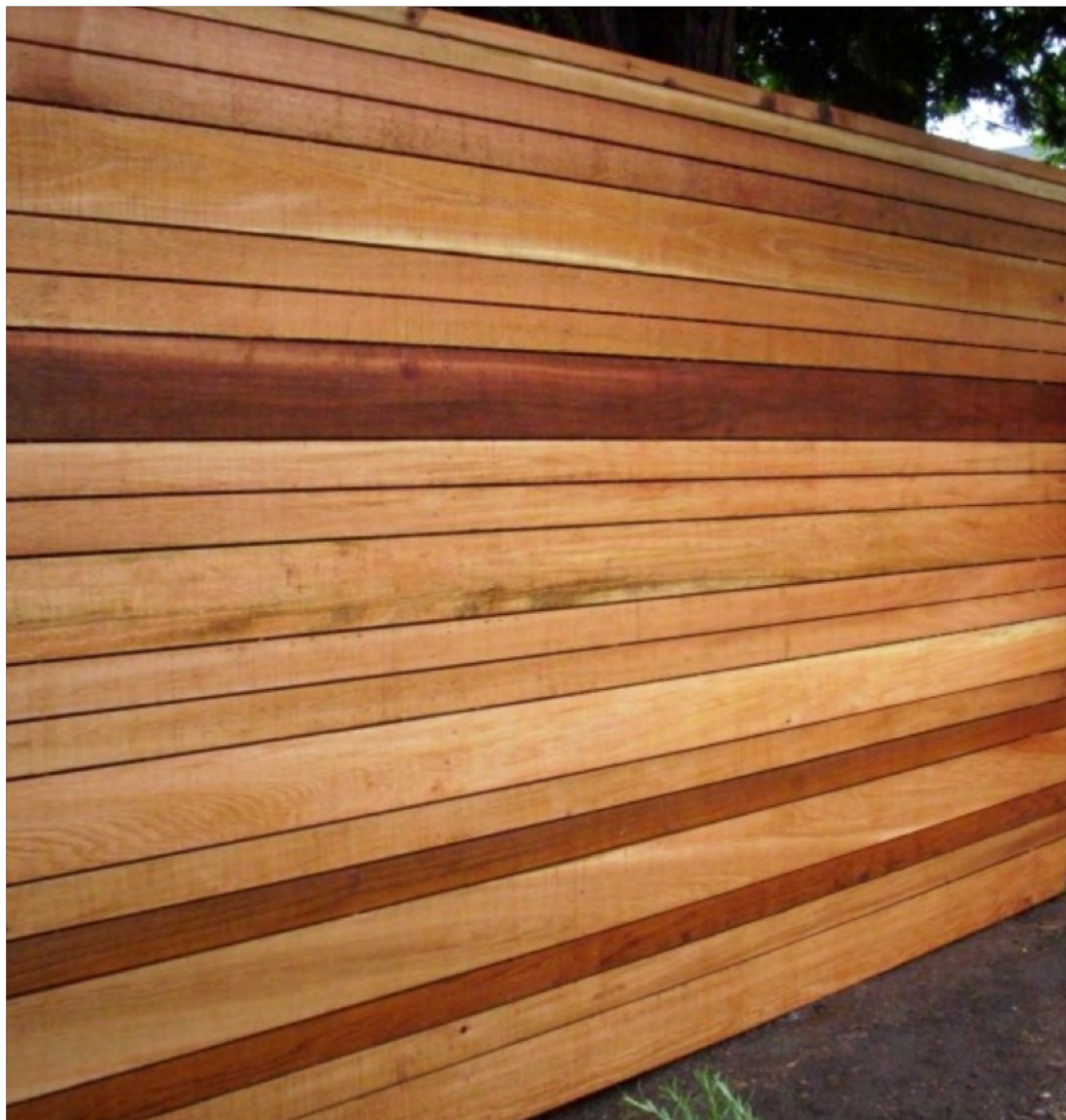
Fencing on Perimeter
