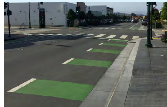
Broadway Avenue road diet in Seaside, CA
