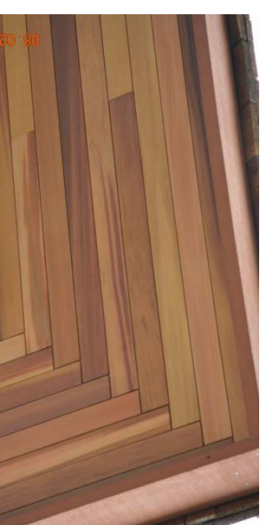
Cedar accent wall and soffits
