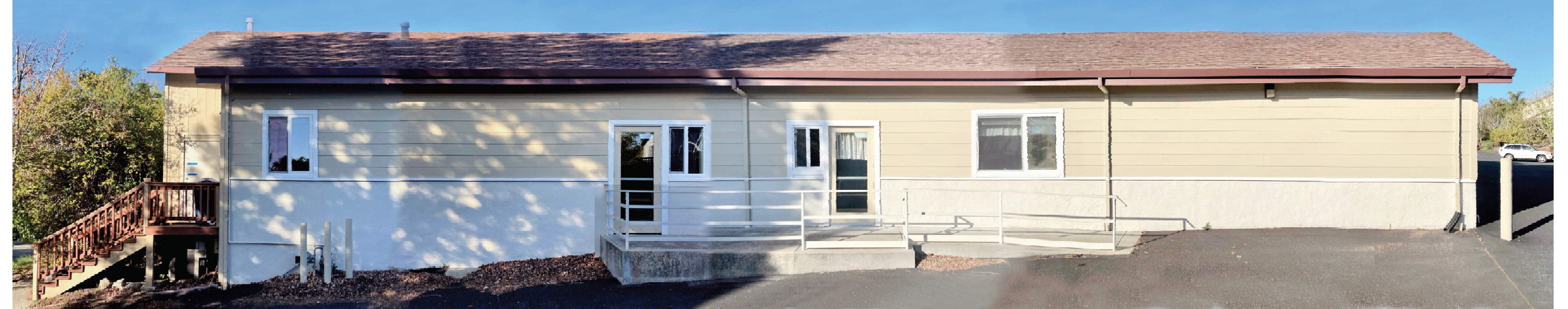
3 South West Facade (No Change)
