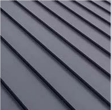
4 Standing Seam Metal Roof
