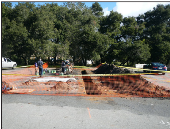
Photograph 5. Crew dry screening soils (facing east).
