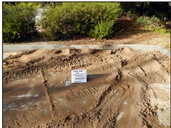
Photograph 6. Trench 2 backfilled after collapse (facing north).
