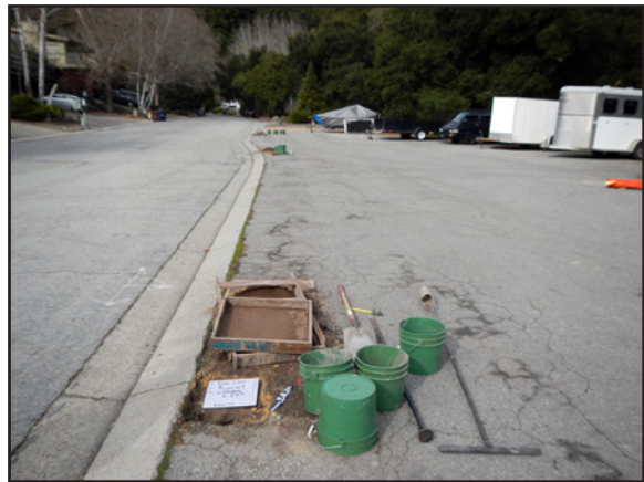
Photograph 4. Overview of augered areas (facing north).
