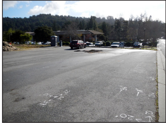
Photograph 2. Trench 4 backfilled (facing southeast).
